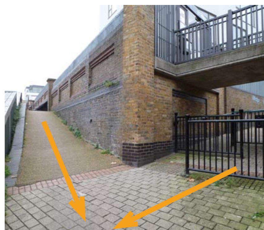
6 Hazardous pinch points
