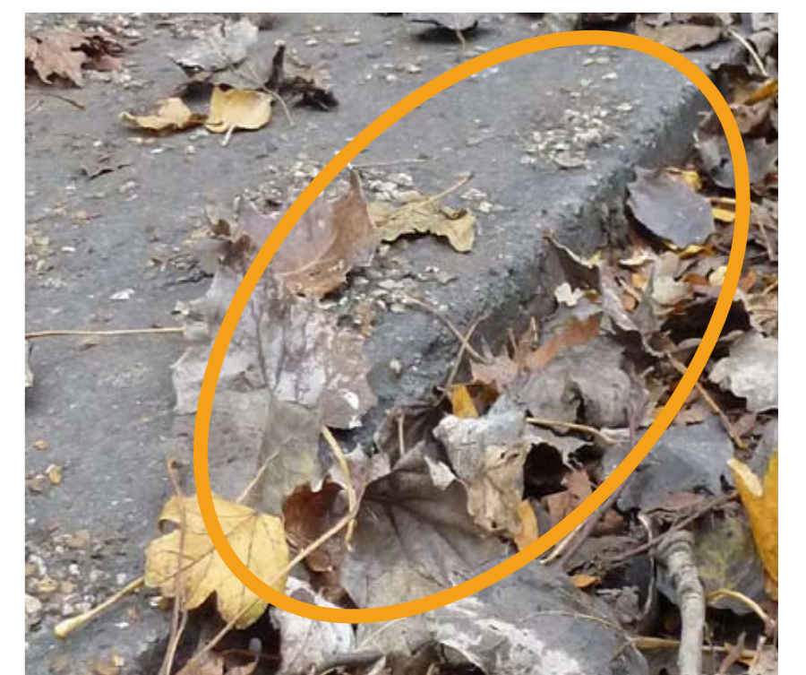
4 Trip hazards caused by worn areas in the grass verges.
