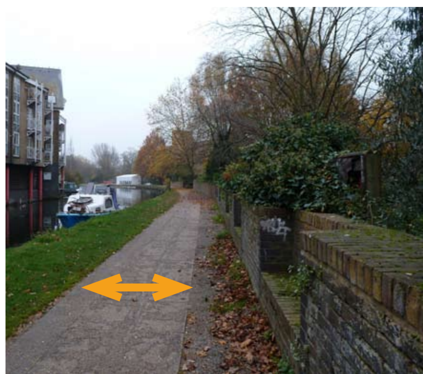
1 Narrow towpath allows limited space for cyclists and pedestrians to pass safely.
