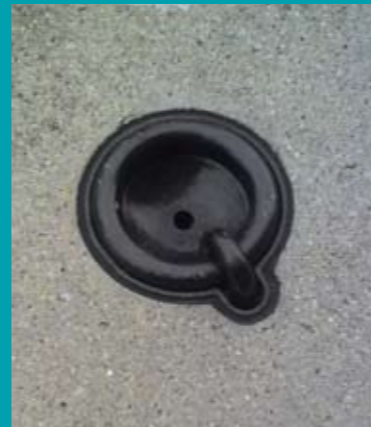
Repair/replace copings and add mooring rings
