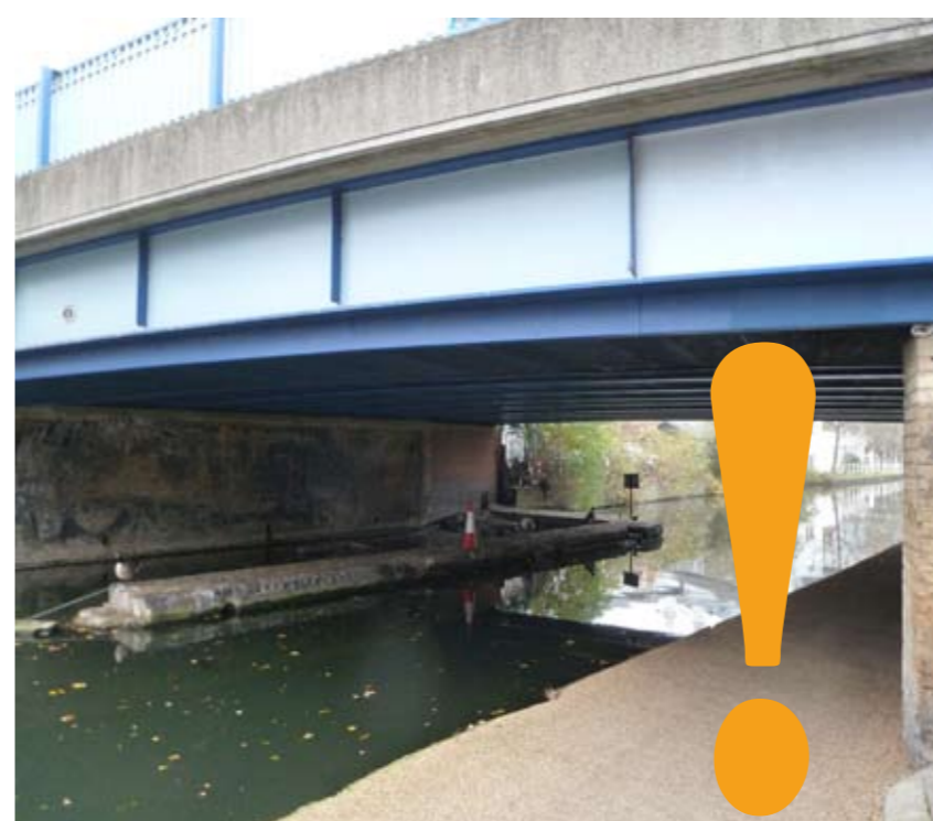
7 Blind spots at access points and bridge holes
